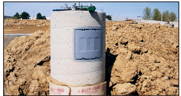
2. Remove form after concrete has been poured and allowed to cure.
