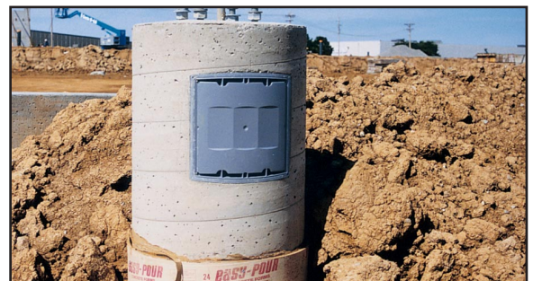
4. After wiring is completed, the lid is replaced to complete the installation.
