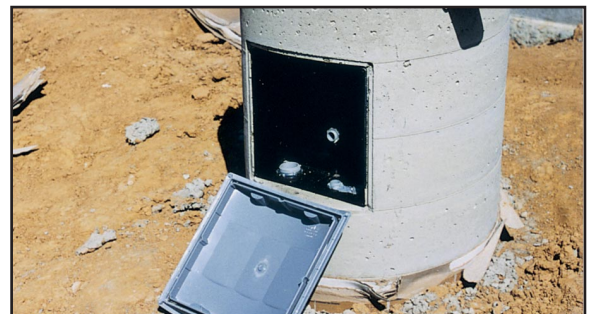
3. Pop off the J-Box lid, leaving an 8" x 8" x 4" or 12" x 12" x 4" access area, depending on the J-Box selected.
